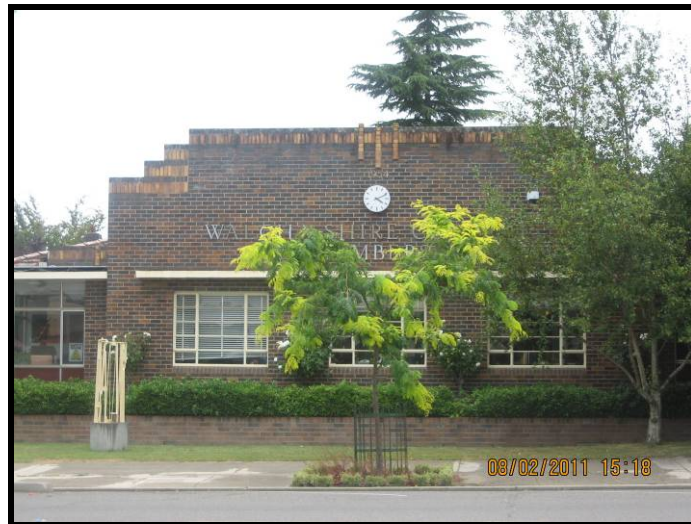
Walcha Council Chambers
