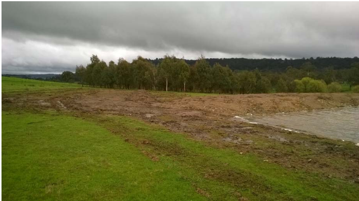
Completed earthworks to raise the dam wall.
