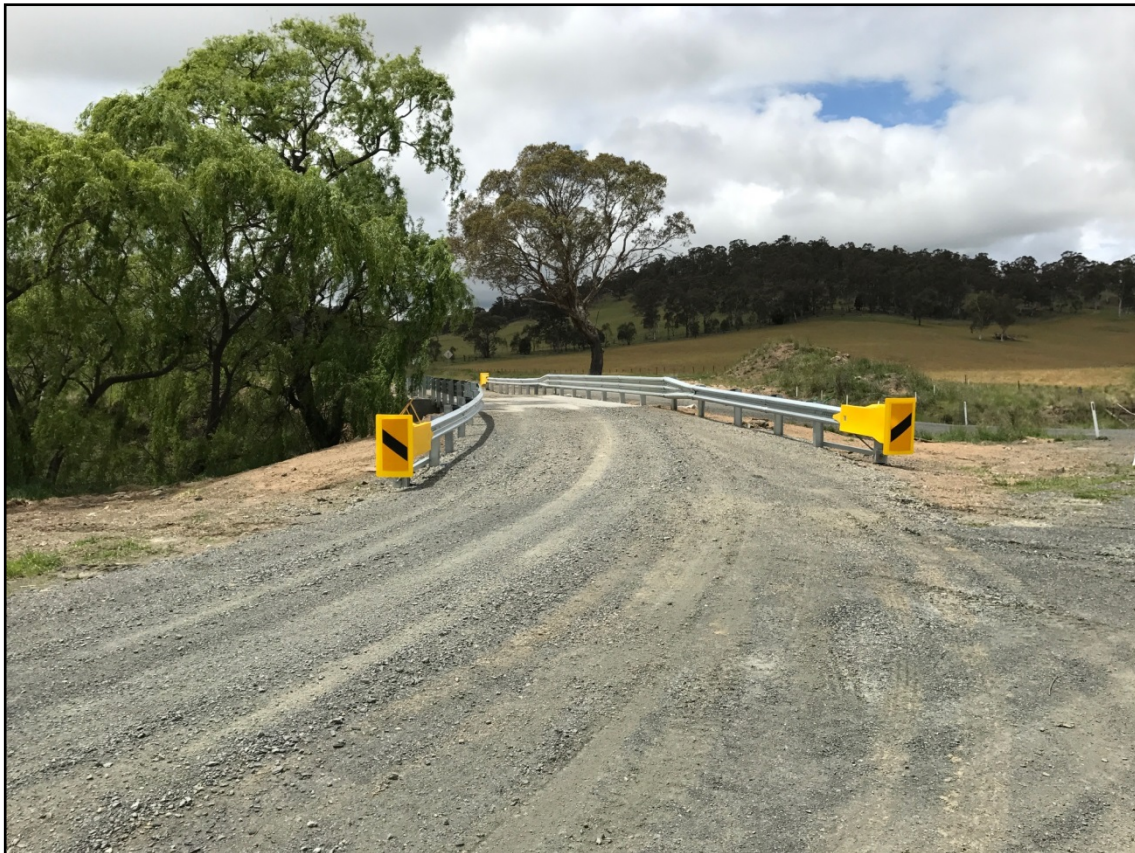
Hartford Road bridge
