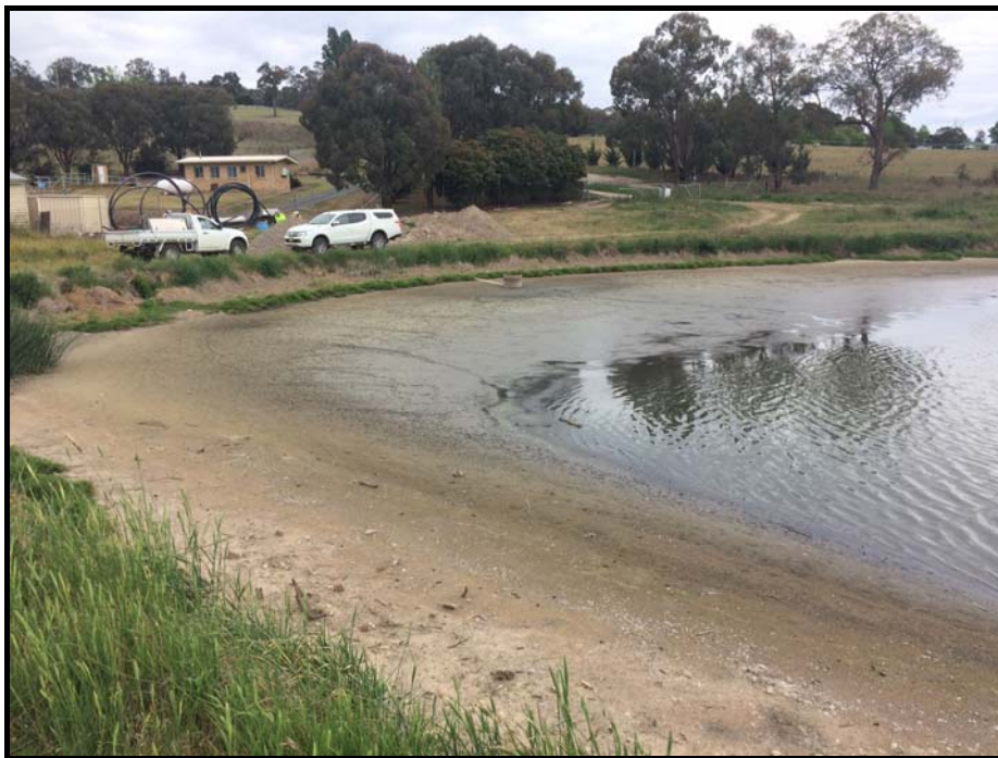
Photo showing exposed sludge and the water level dropping in the maturation pond.
