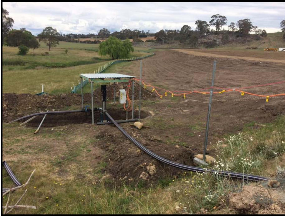
Temporary pump station for the emptying of the maturation pond.
