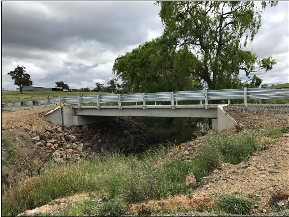
Hartford Road bridge – Number 2
