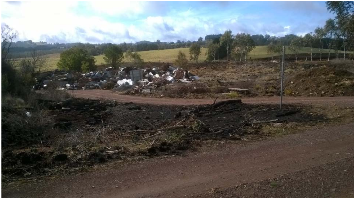
Landfill site before the earthworks
