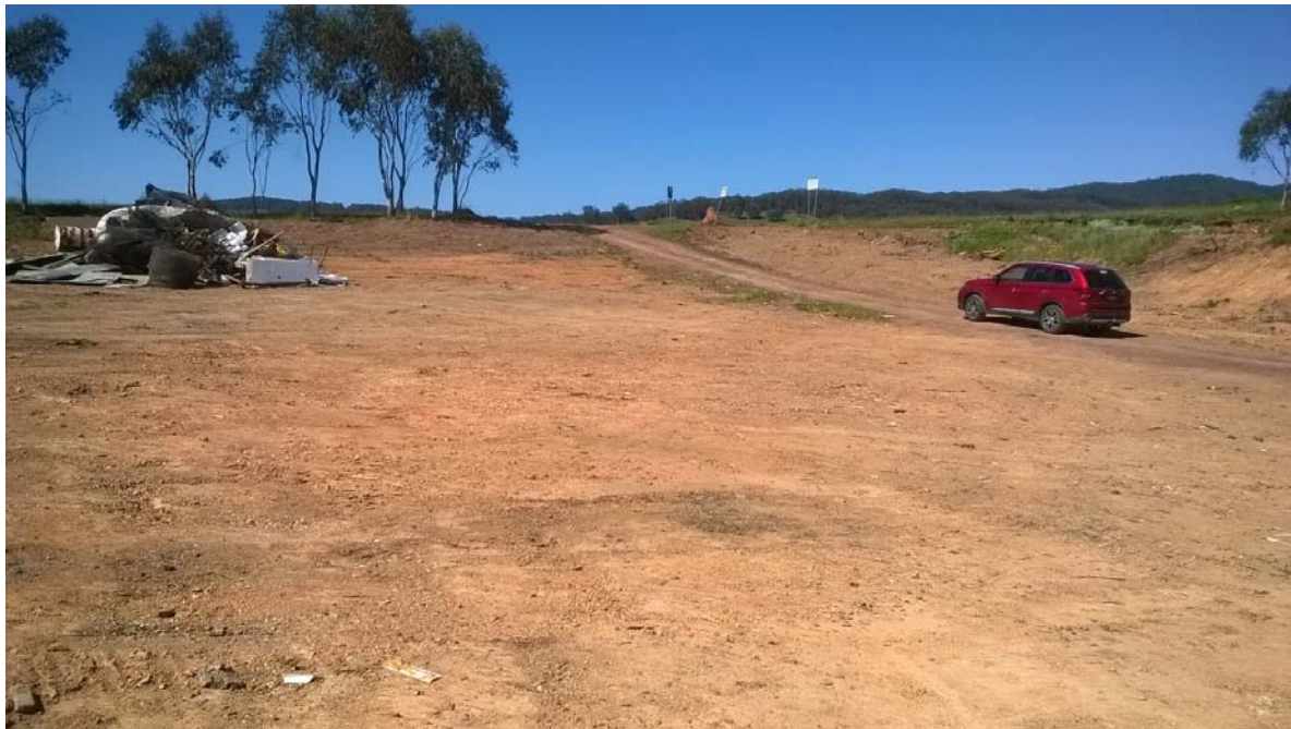
Landfill site after the earthworks
