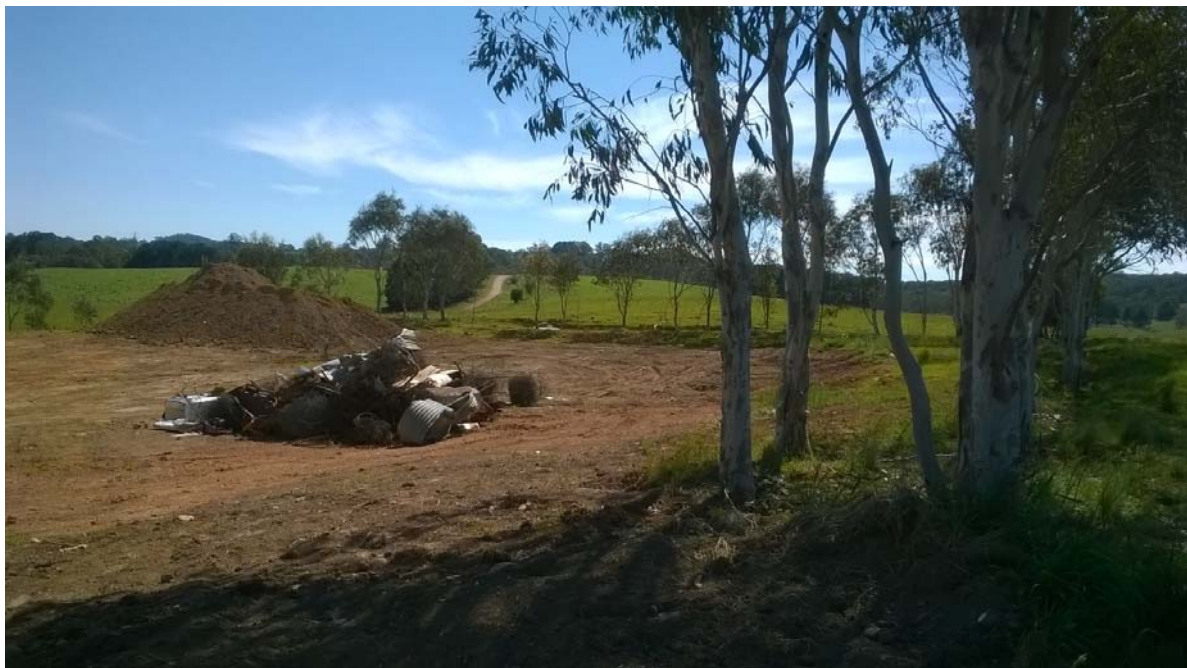
Landfill site after the earthworks
