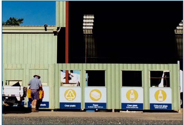
Figure 1 - Recyclables separation windows at the WWF
