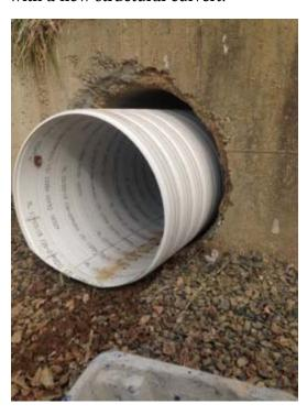
This means that the road doesn't need to be excavated or disturbed, saving great deal of money on culverts that are located deep beneath the road surface.
