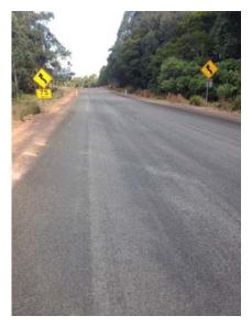
and potholes were the general problems with these patches. However, stabilisation and recompacting has led to good results. The seal may tend to strip or break-up due to being installed in cold weather, which will be closely monitored.
