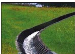
The final stage of the Jamieson street rehabilitation is the placement of Smart-Ditch drainge between middle street and Brian Smith Timer Tansport. Smart-Ditch has been installed to improve erosion and sediment controls, convey water more efficiently and improve the aesthetics of the road.
