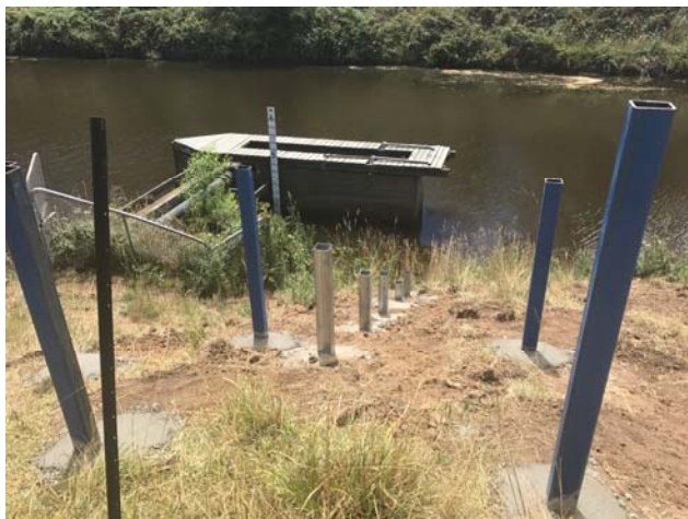
Photo below of piles/supports for the last of the pipework that extends down to the pump housing in the River. New pipework running to the dam in photo on the right.
