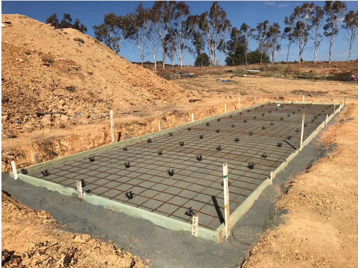
Form work for the new general waste skip bin.
