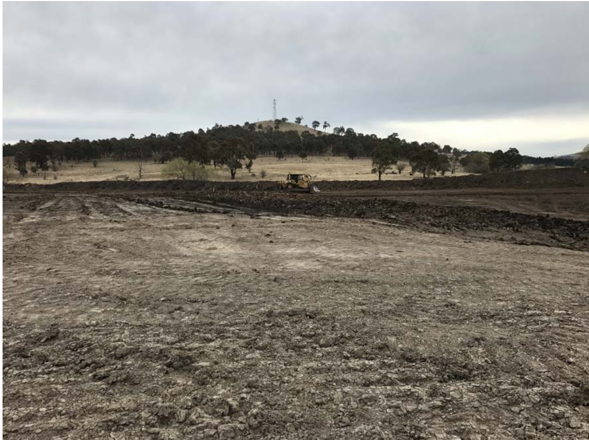
View to north (Sugarloaf Hill).
