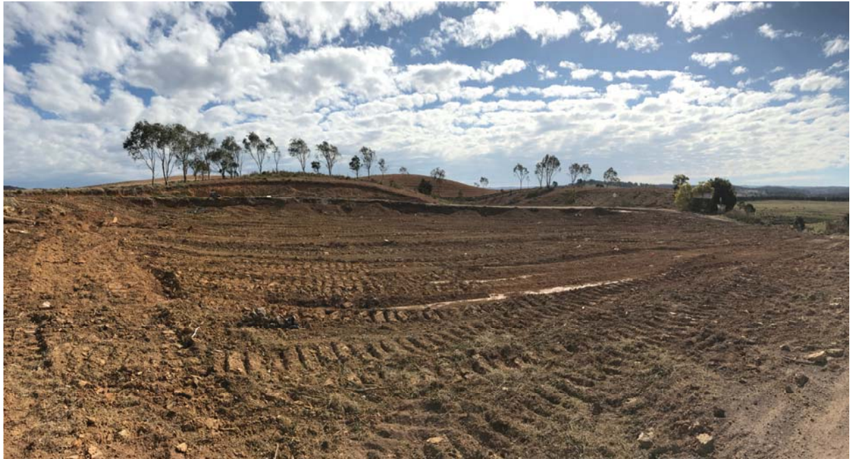
Old landfill cell backfilled.
