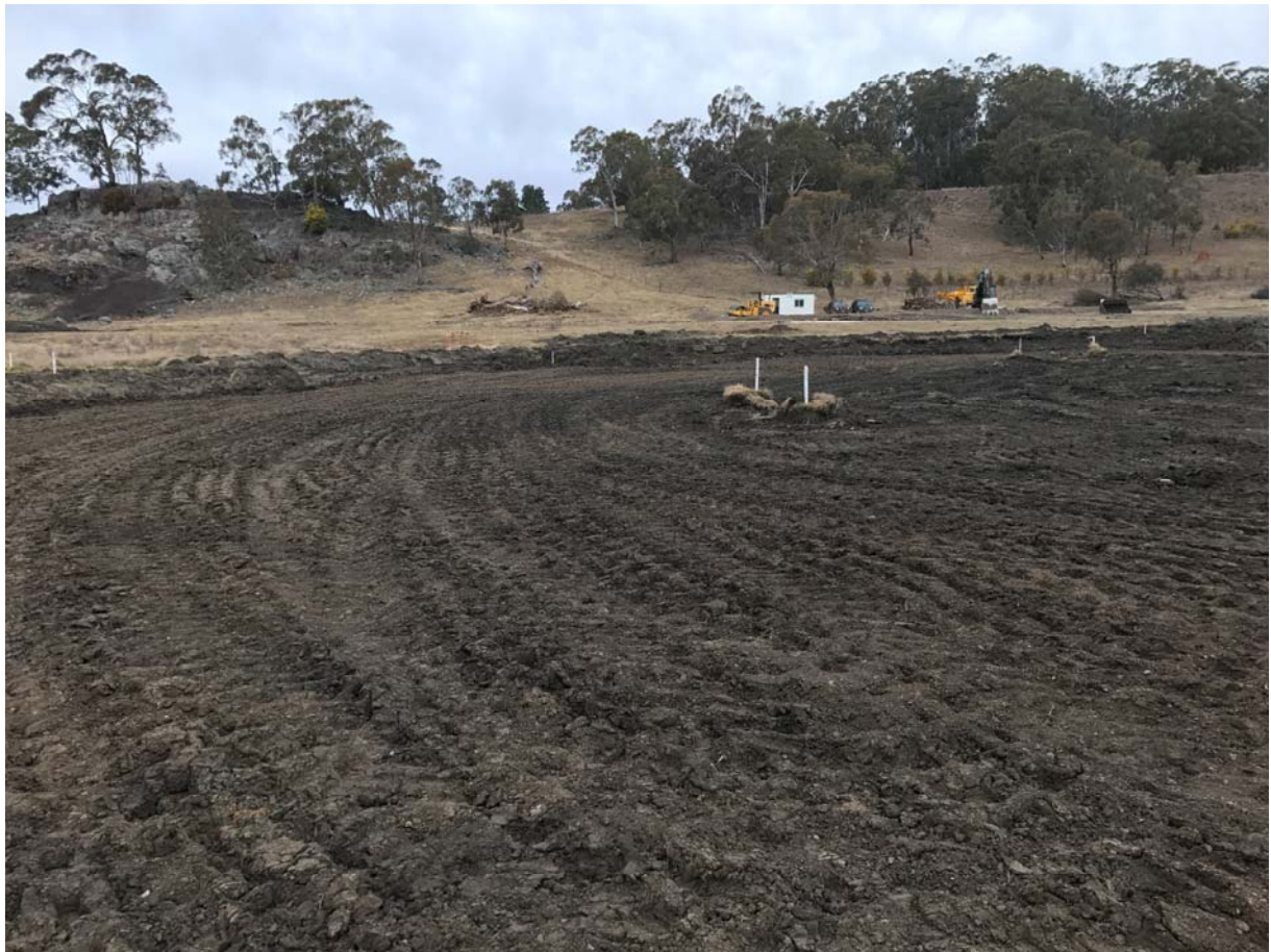
Stripping of grass/top layer.
