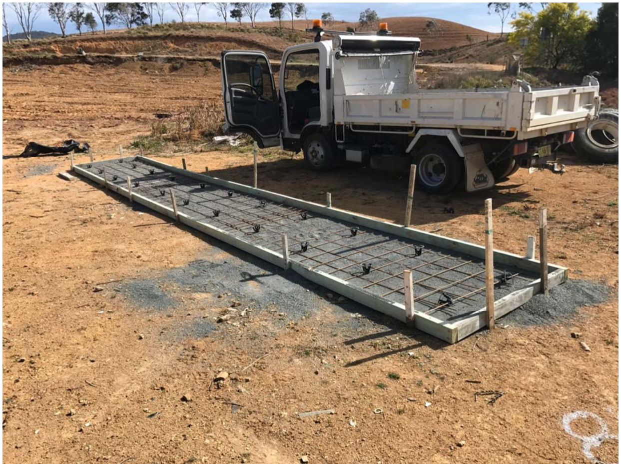
Form work for the new recycling corrals.
