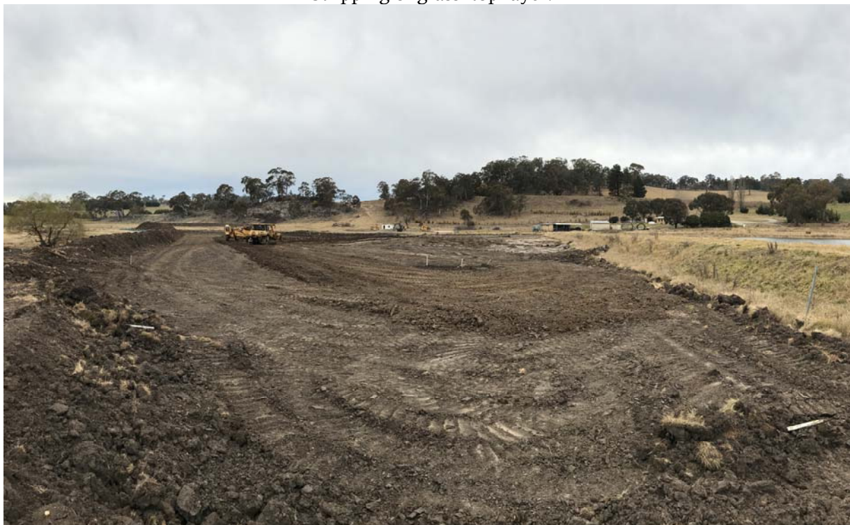
Showing adjacent maturation pond wall to right of photo.
