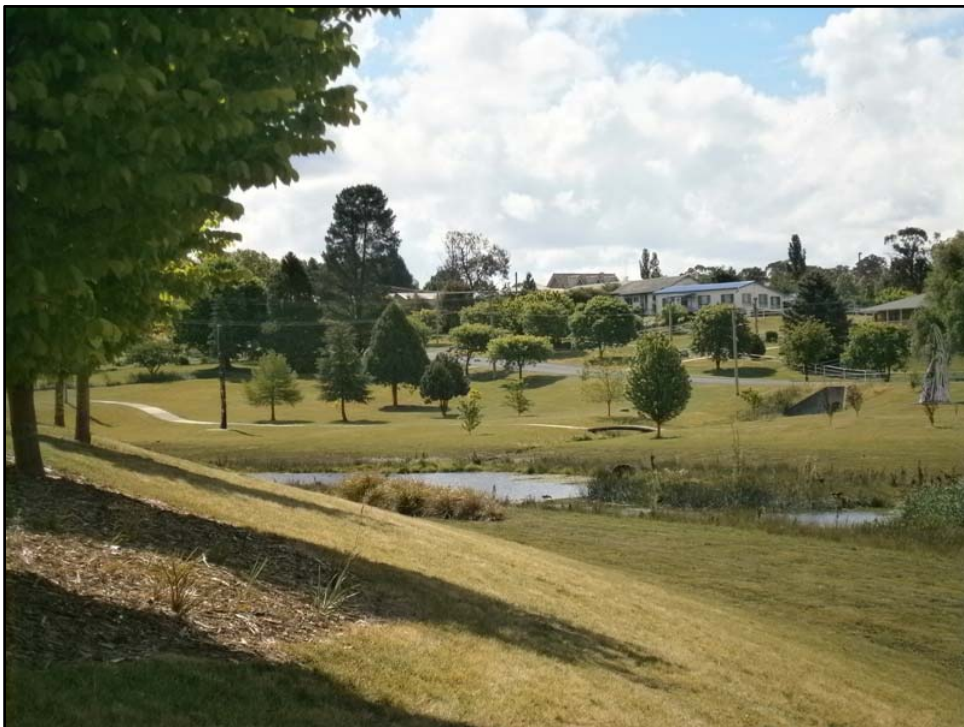
Apsley River Levee Banks
